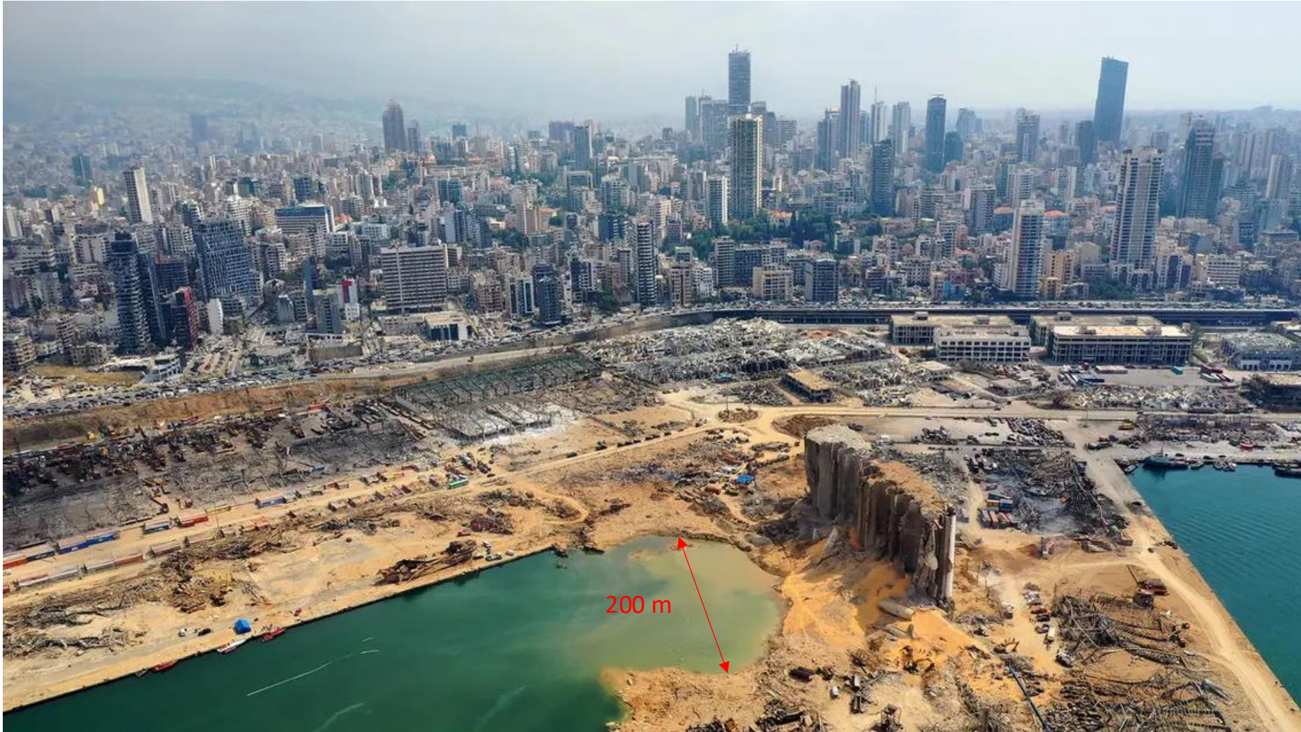
Beyruth 2020: Explosion of 2 750 tonnes ammonium nitrate stored in shed.
